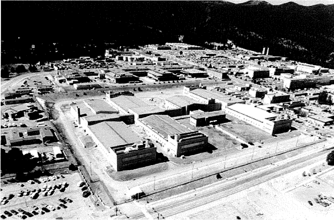
Figure 2–1 Existing Chemistry and Metallurgy Research Building
