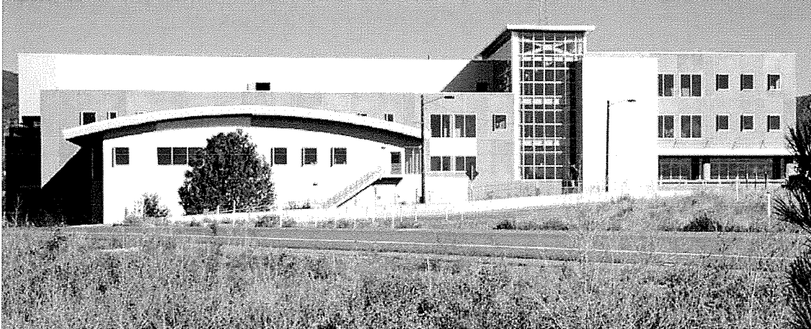
Figure 2-3 Radiological Laboratory/Utility/Office Building in Technical Area 55
