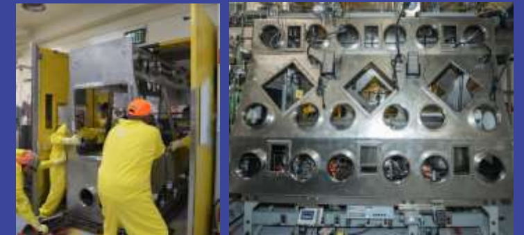
Transfer and install in the Plutonium Facility
