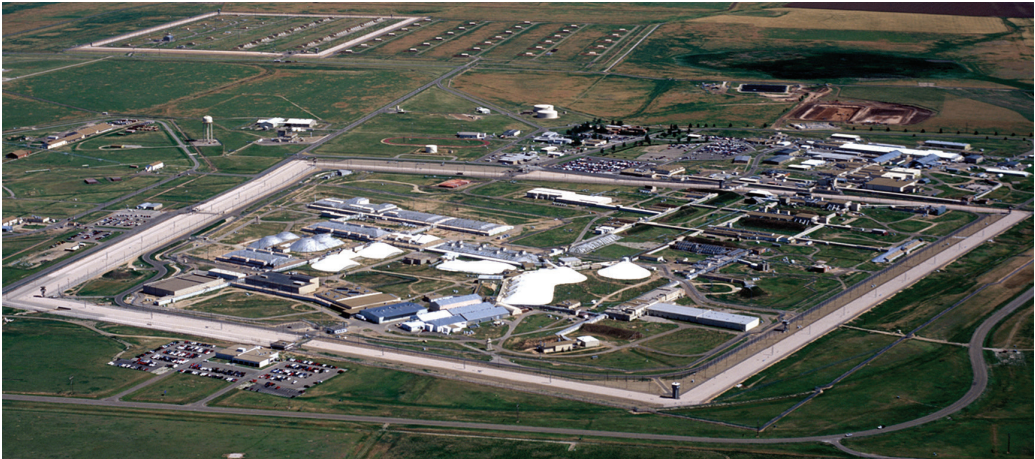
Figure D.4 Pantex Plant
