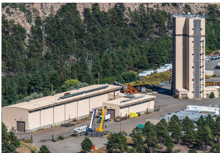
Figure 14.2 LANL Rack Assembly and Alignment Complex (RAAC)
