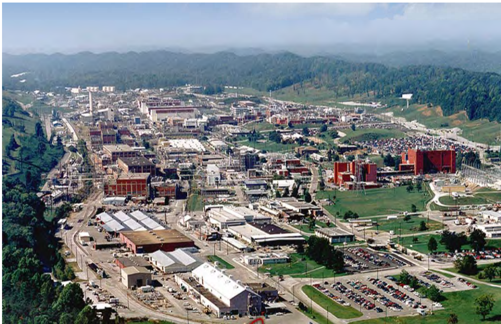
Figure 1 The Y-12 National Security Complex
