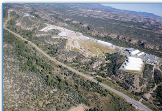
TA-54, as seen from the air, contains numerous sprung-structure domes storing TRU waste awaiting shipment to WIPP.
