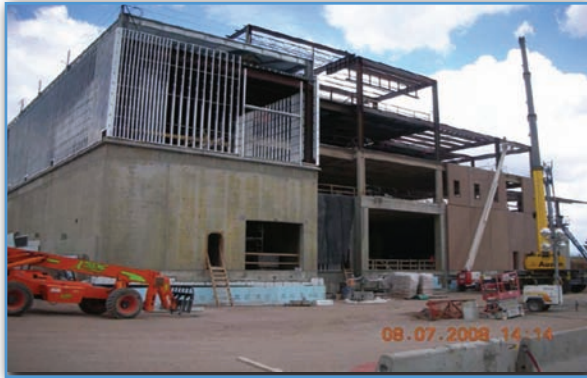
The completion of the CMRR project, currently under construction, will contribute to the Laboratory's nuclear facility consolidation efforts.
