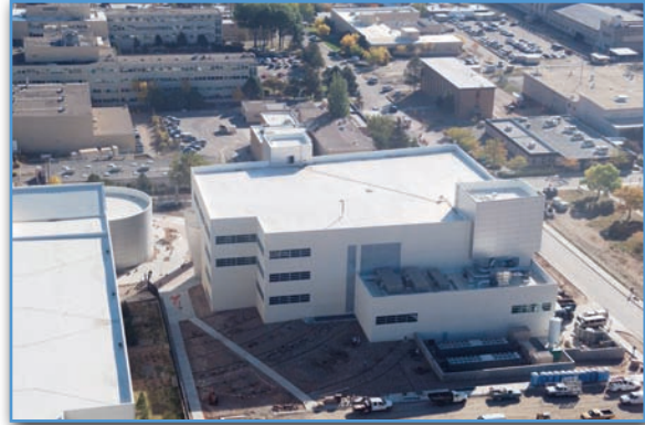
Although the NISC is a notable exception, many of the structures that support Threat Reduction are old and deteriorating.
