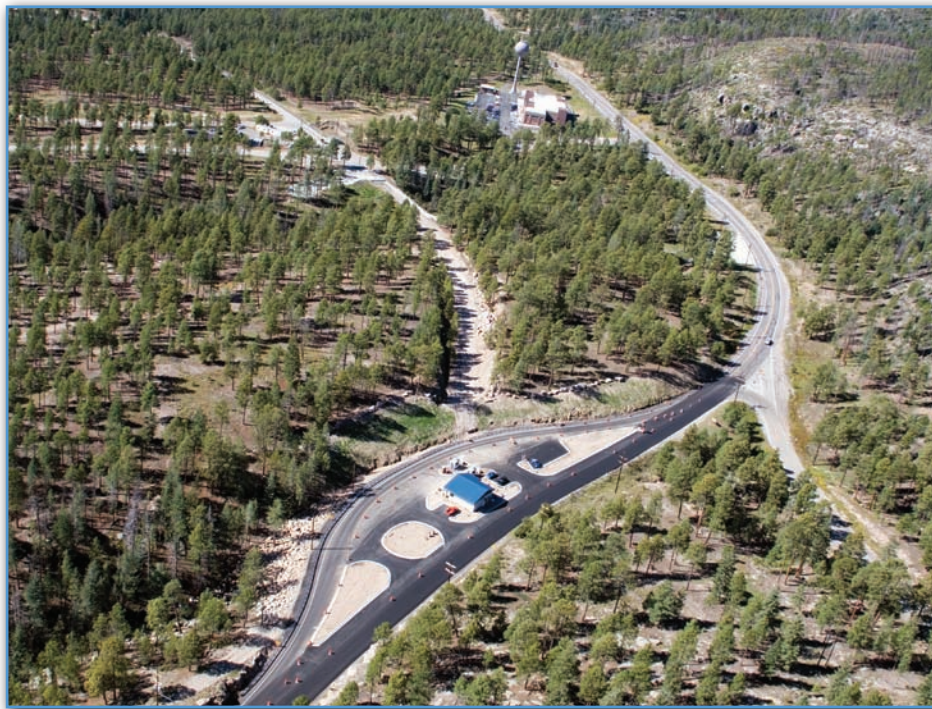
Security enhancements such as the Security Perimeter Project completed in FY07, provide the site with a high level of protection for existing Laboratory assets.
