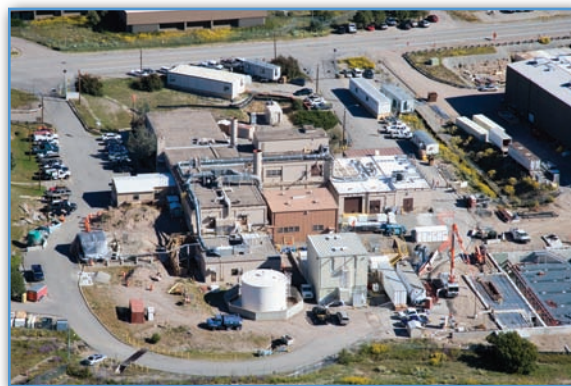
The RLWTF upgrade will enhance reliability and process capability to meet projected regulatory requirements for discharge.
