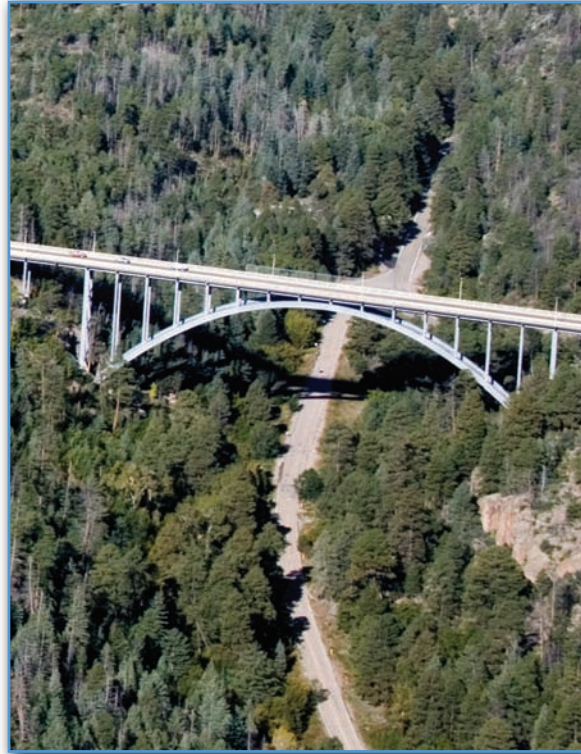
The Omega Bridge, constructed in 1951, is in need of significant maintenance within the next ten years due to deterioration of the concrete decking and seismic compliance concerns.
