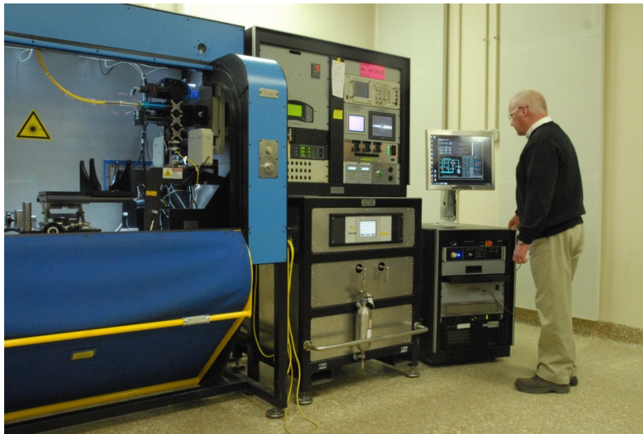
Fig. P12. Laser gas sampling station.
