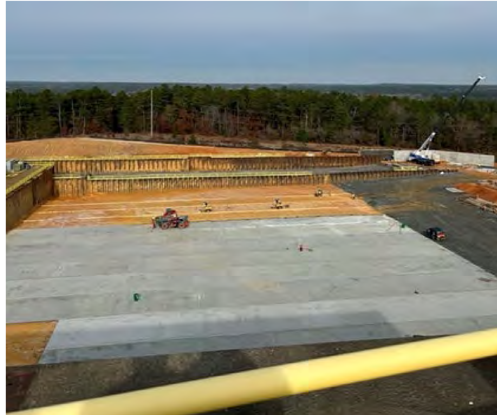
SRPPF project ongoing construction of the sand filter
