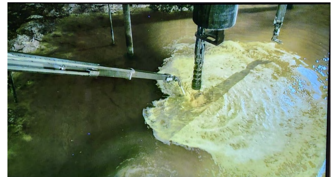
Retrieval of liquid high-level radioactive waste at the Hanford Tank Farms
