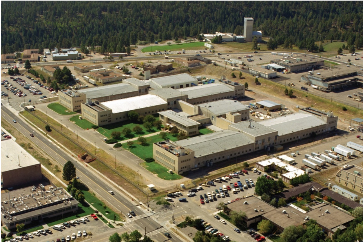
Figure 2-2. The CMR Building at TA-3
