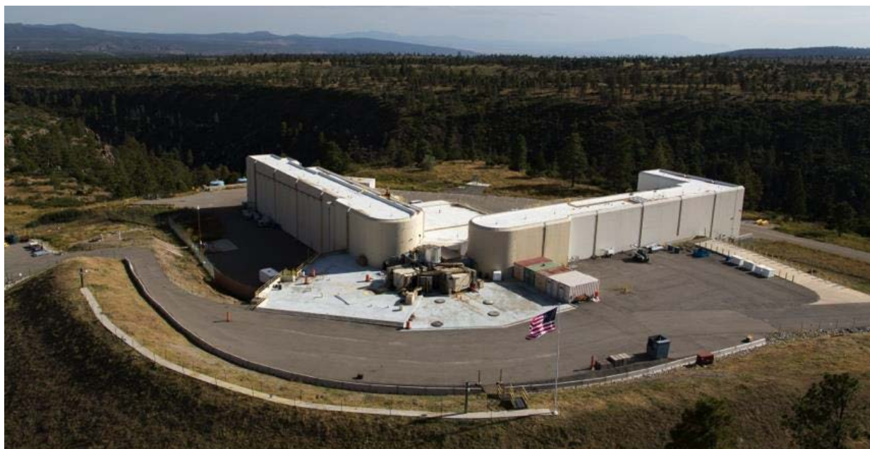
Figure 2-5. The DARHT Facility
