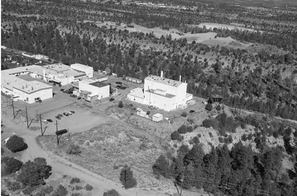
Figure J-7 Photograph Looking North Across Mortandad Canyon in the Area of the Bridge for Proposed Auxiliary Action A
