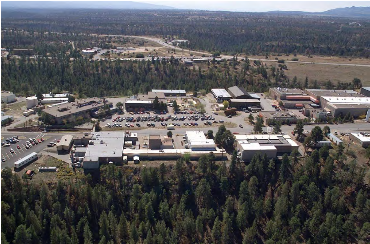
Figure J–5 Photograph of Canyon to be Bridged between Technical Area 35 and Technical Area 63
