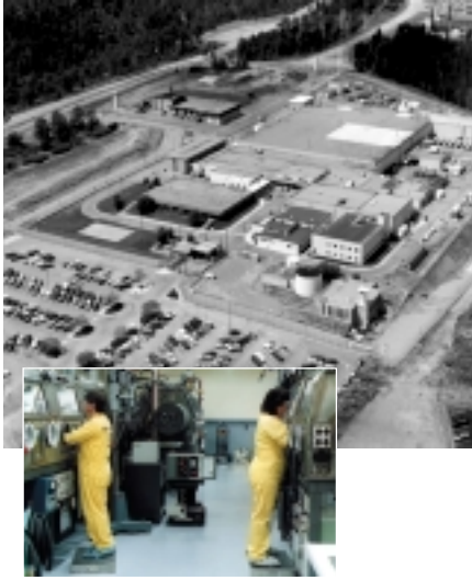
The plutonium facility at Los Alamos is developing the capability to remanufacture small lots of plutonium pits and now carries out all surveillance activities necessary for stockpile stewardship. All experiments and tests are conducted inside a glove-box environment (inset).
