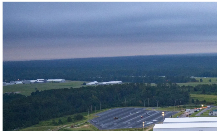
Full construction can now begin at the Savannah River Plutonium Processing Facility (SRPPF) at the Savannah River Site.
